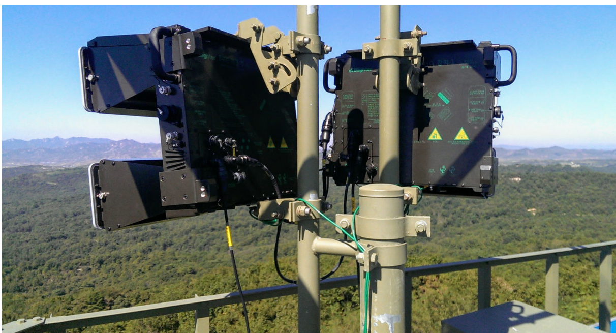
Figure 5: Blighter B400 series radar installed on Korean DMZ
